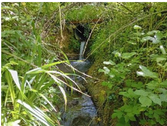
Figure 11: Stream emerging from culvert pipe at north.
